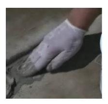
Place material in the cracked area. This will help ensure a good bond.
