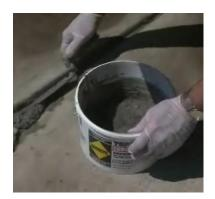
Add additional dry material to the mix to increase the consistency. Using a margin trowel, add more product to the damaged area.
