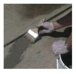
Apply the finishing touches to the area using a paint brush to blend the Top N Bond material to the existing concrete.
